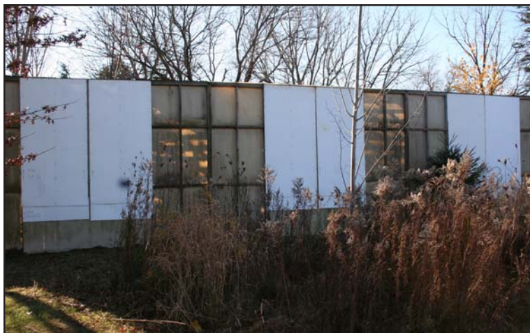
Short-eared complex after winter paneling installed
