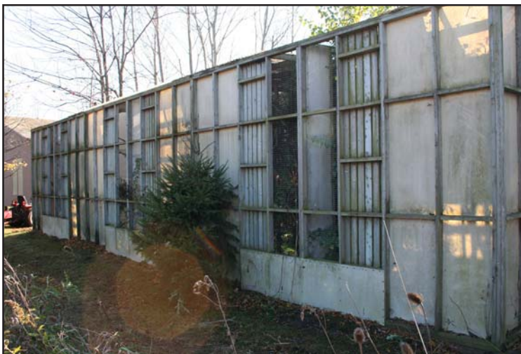
Short-eared complex before winter paneling installed
